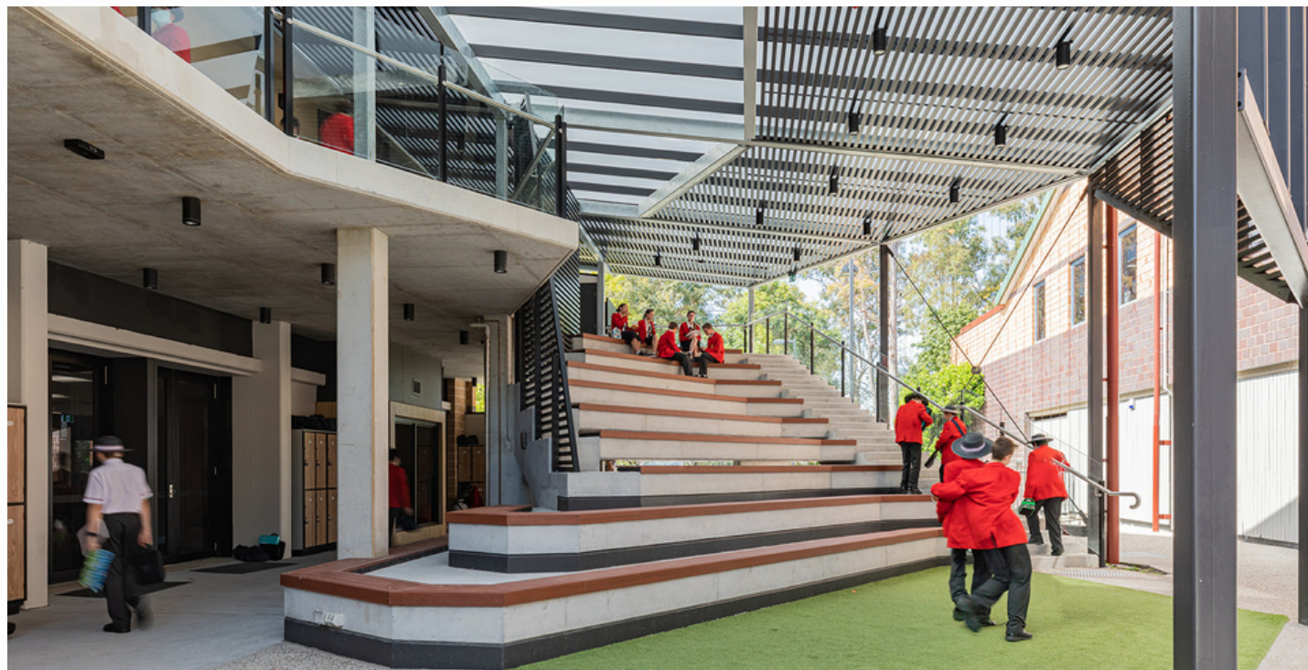
Image: 2023 LEAD Awards Winner of Category 5: Modernisation, Large - All Hallows' School - The Potter Building Adaptive Re-Use Project, Queensland, Australia | ARCHITECT: Fulton Trotter Architects | PHOTOGRAPHER: Scott Burrows
